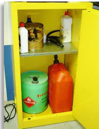
This flammable liquid cabinet is designed and built in accordance with Underwriters Laboratories (UL) 1275, Flammable Liquid Storage Cabinets .
